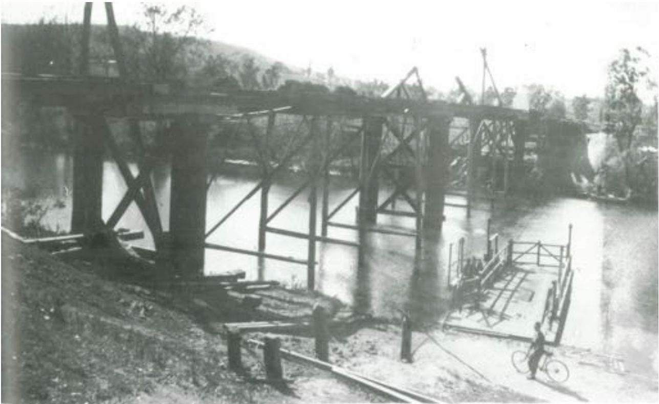
Figure 11: Construction of the New Bridge with river punt, circa 1878–1879. It is not clear whether the photograph was taken before or after the August 1879 flood. From RL Ford, Clarence Town: Erring-I to river port, p 223.
