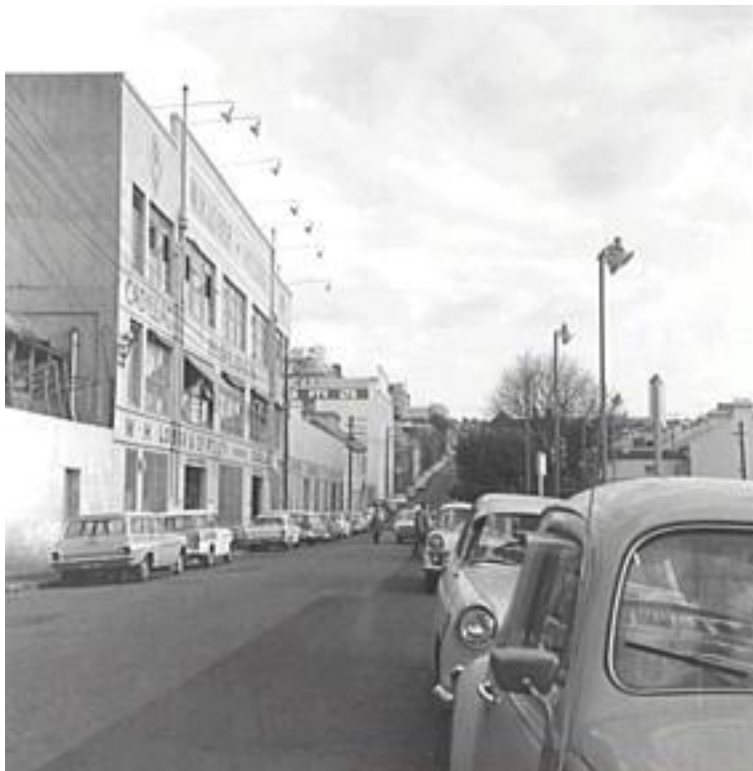
Figure 11: View S from Pring St of Eastern side of McElhone St. WH Lober and Co Motor Vehicles on L. 23 August 1968, SRC8085. Originally from file 0864/68 (CRS 144). City of Sydney Archives.
