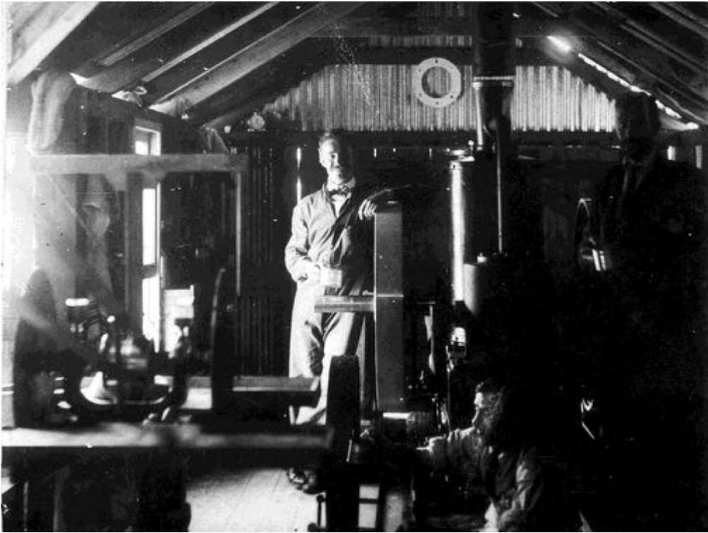
Figure 45: Engine room, Wallabadah station. This image shows the steam engine. SLNSW, bcp_04073
