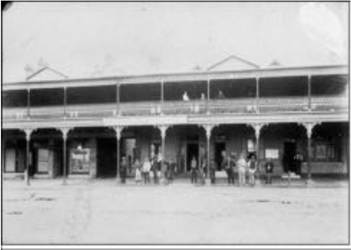
Figure 9: Commercial Hotel, George Street Quirindi with a second storey added in 1895. The building was extended over the carriageway in 1901, creating three small shops. The over footpath verandah has been removed. K Halliday and Liverpool Plains Shire Heritage Community Advisory Committee, Community Based Shire Wide Heritage Study Documents 2004-05
